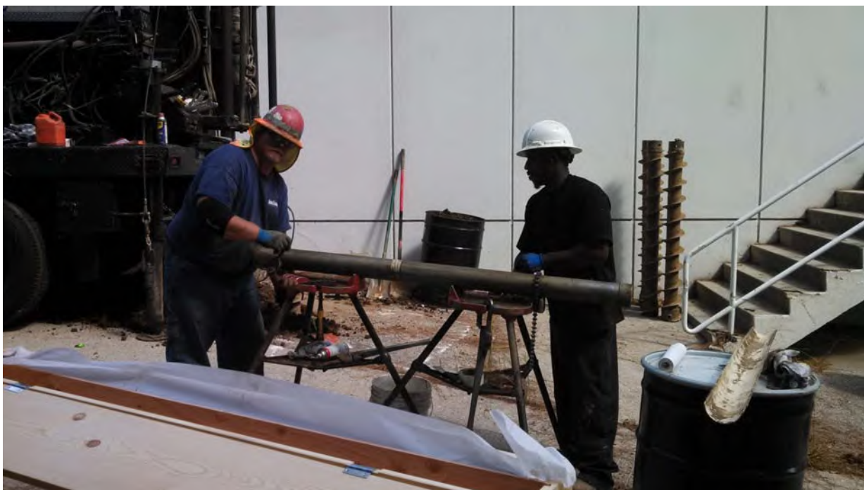
Photo 10: Core barrel retrieval
