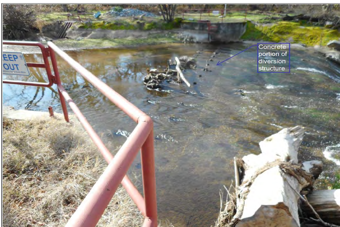
Figure 11c. Hemphill Diversion Structure Flashboards Not Installed
