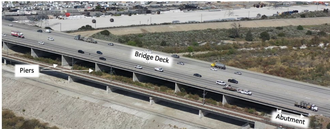
Figure 1.1-d. Image of I-210 San Gabriel River Bridge with Typical Bridge Components Labeled
