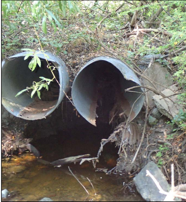
Photograph 3. Photograph taken of degrading culvert outfalls proposed for replacement in Cherry Creek. Photograph taken July 31, 2017.
