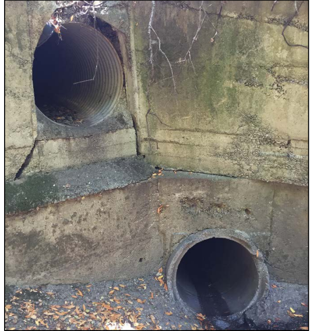
Photograph 4. Photograph taken of inlet hi/low culverts northwest of Sandra Road. Photograph taken July 31, 2017.
