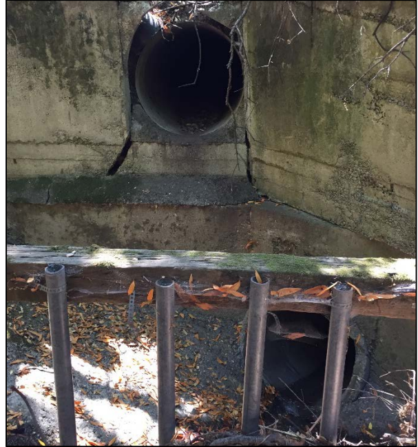
Photograph 4. Photograph taken of inlet hi/low culverts and trash wrack northwest of Sandra Road. Photograph taken July 31, 2017.
