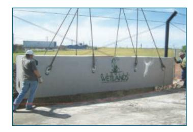
The Modular Wetlands® is simple, easy to install, and has a space-efficient design that offers lower excavation and installation costs compared to traditional tree-box type systems. The structure of the system resembles precast catch basin or utility vaults and is installed in a similar fashion.
