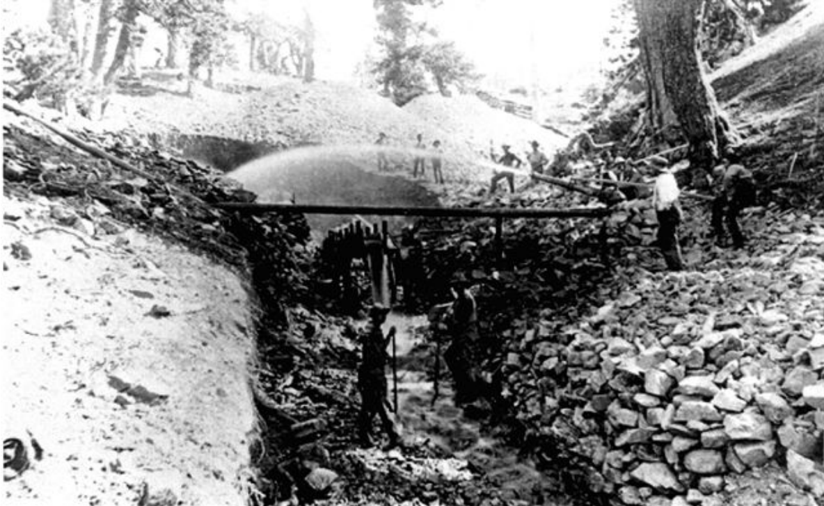
Figure 3.3-2. Hydraulicking, n.d. Courtesy California Gold Mines, A Sesquicentennial Photograph Collection, California Department of Mines and Geology.
