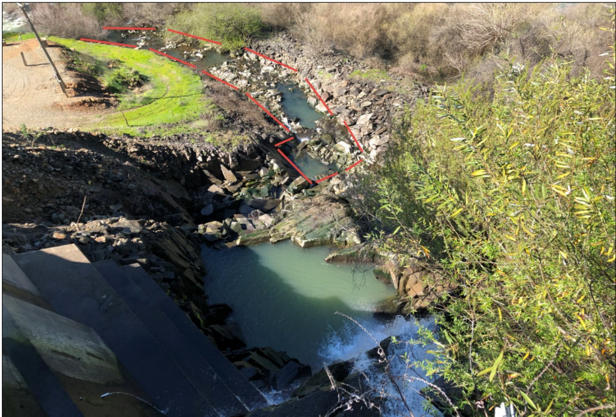
Figure 6. Sluice channel from above with proposed shotcrete boundary
