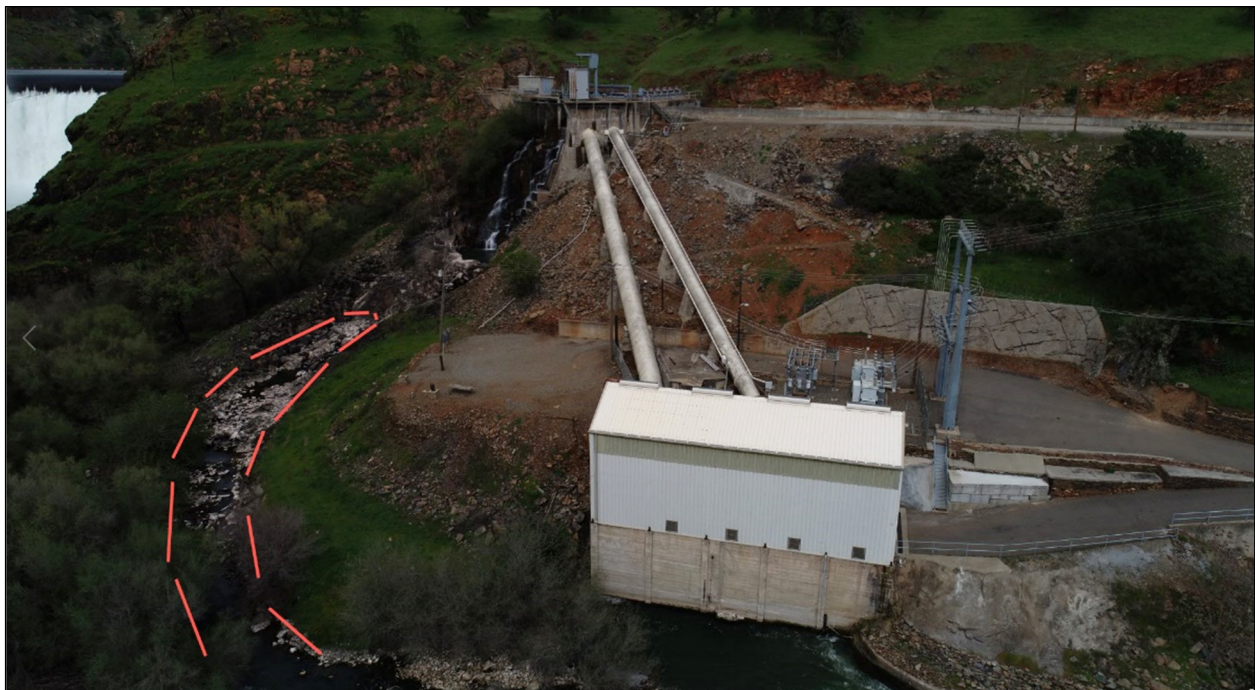
Figure 4. Sluice channel proposed shotcrete boundary
