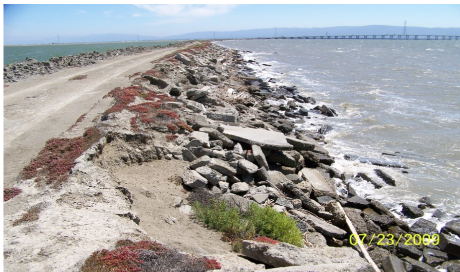
Figure 2-6. Riprap Placed on Outboard Side of Berm
