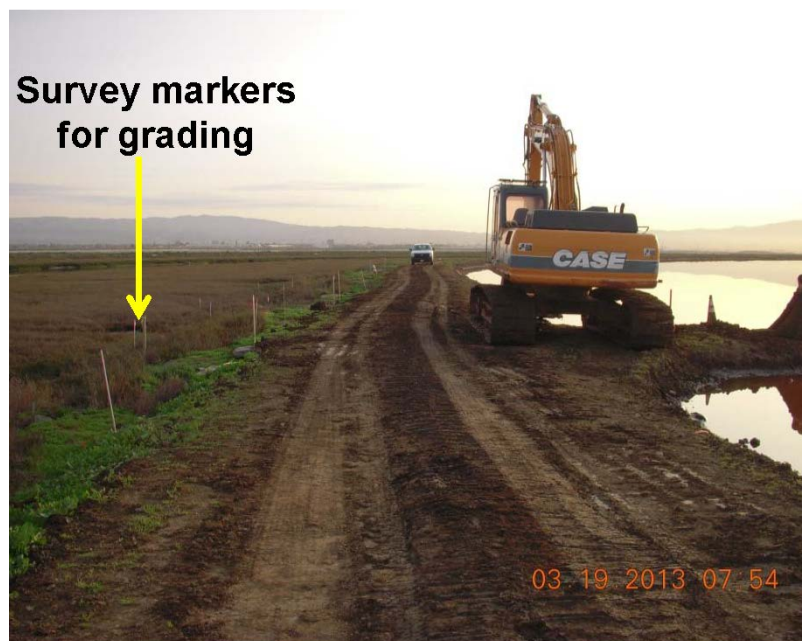
Figure 2-4. Example of Stakes Being Placed to Set the Grade Level
