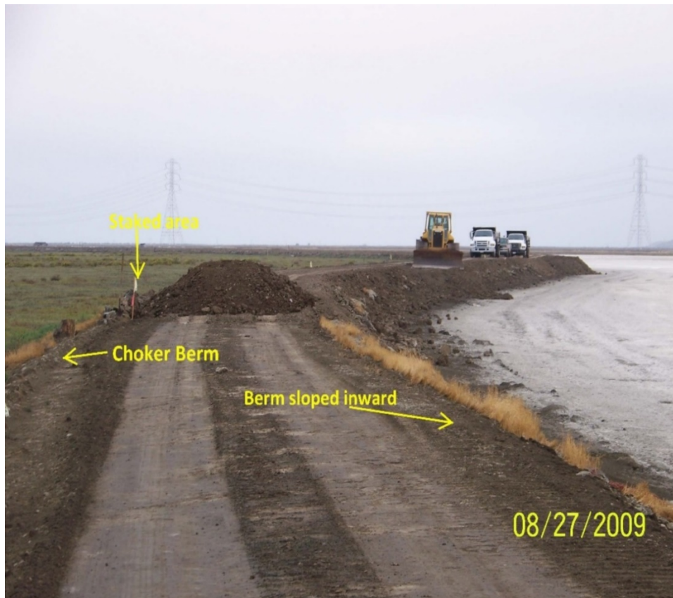
Figure 2-2. Example of Choker Berm and Inward Slope on Berm
