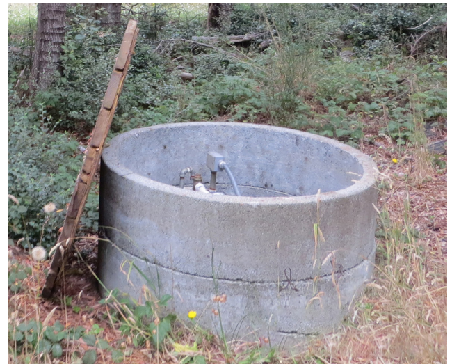
Well #2 Concrete Caisson Enclosure with Wood Lid
