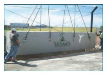
The Modular Wetlands<sup>®</sup> is simple, easy to install, and has a space-efficient design that offers lower excavation and installation costs compared to traditional tree-box type systems. The structure of the system resembles precast catch basin or utility vaults and is installed in a similar fashion.
