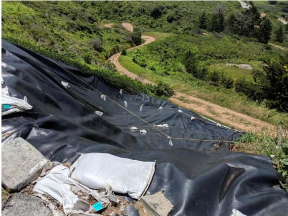
Photograph 1. Project site, looking west towards project staging area and SR 1, showing current temporary plastic tarping for slide control
