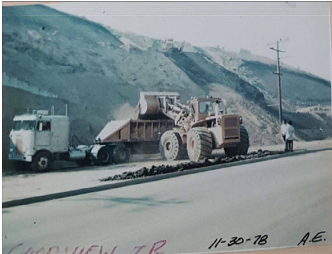
PICTURE 12 (below)- Start of Grading in 1978 with Garvey Slope Retaining Wall Visible on Left
