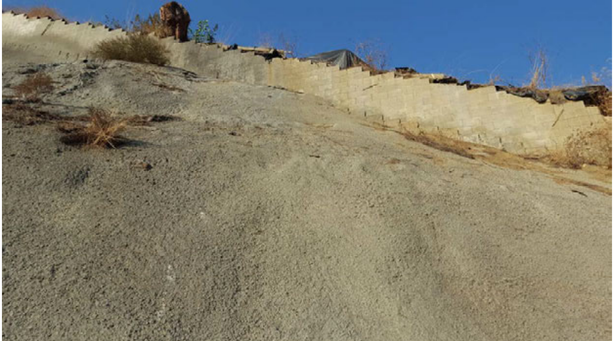
PICTURES 10 and 11 (below)- Abajo Retaining Wall with Shotcrete Slope Below
