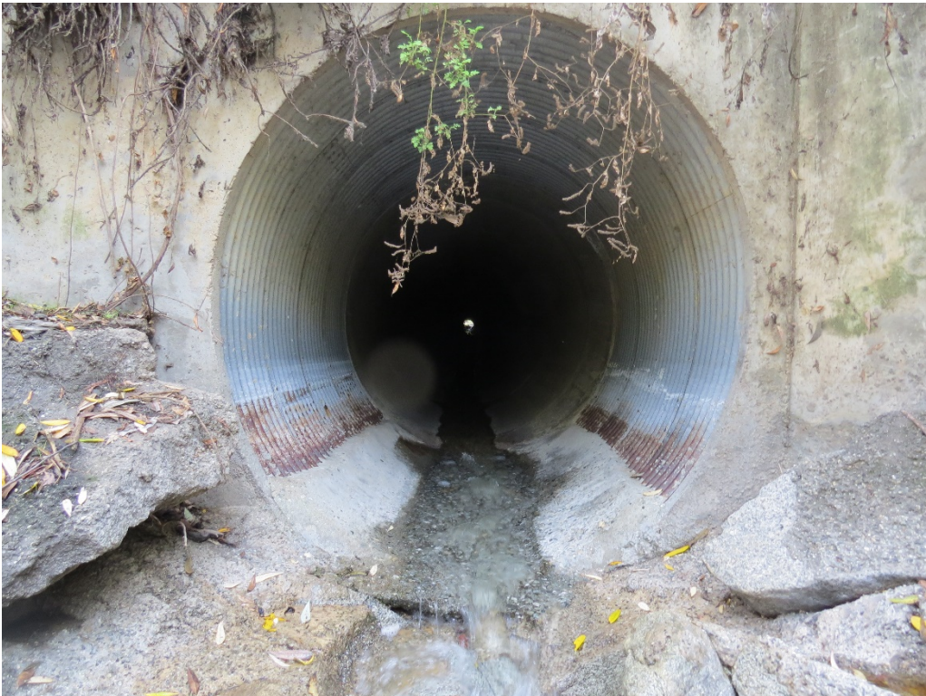
Photograph 8: Looking at the 84-inch culvert under Central Ave.
