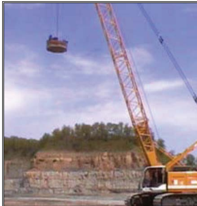
Figure 7-1. Crane Lifting the Tamper
