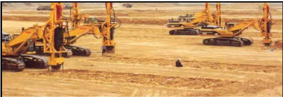
Figure 7-2. Large-Scale Application of Rapid Impact Compaction
