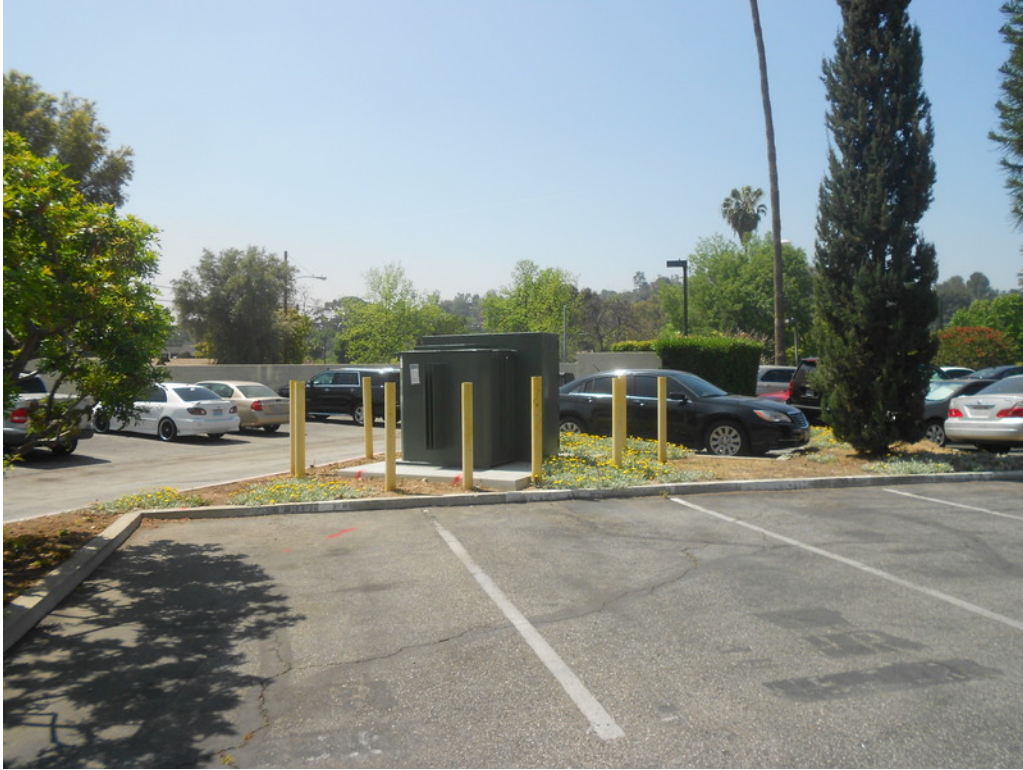
Utility owned pad mounted transformer
