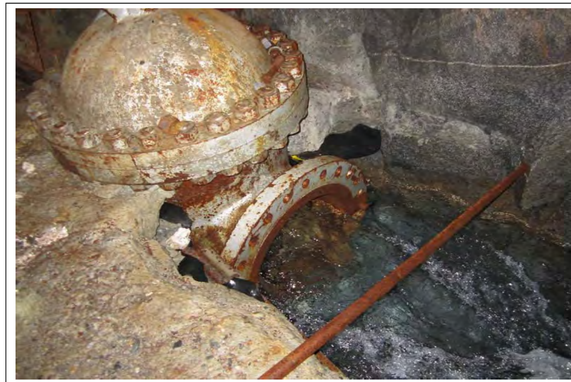
Photograph 8: View depicting water exiting a pipe immediately adjacent to the plug entrance within the Mine tunnel. Photograph taken June 1, 2012.
