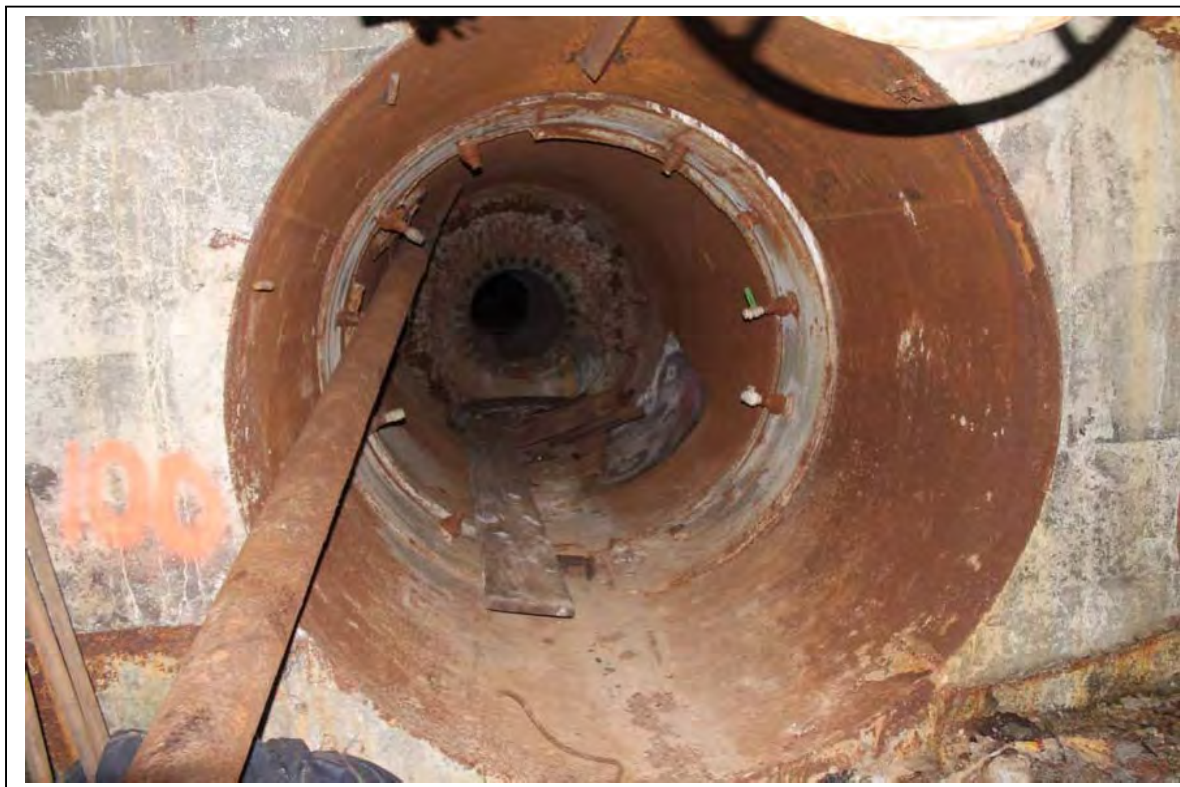
Photograph 7: View depicting the plug entrance (opened) within the Mine tunnel. Photograph taken July 10, 2012.
