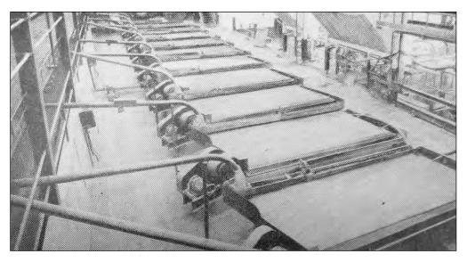
**Figure 15.** Tables separate coarse scheelite for regrinding, and make high-grade concentrate for shipment (Photograph from *Engineering and Mining Journal*, May 1951:83.)
