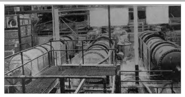
**Figure 16.** Chemical Plant makes pure tungsten and molybdenum products from concentrates. These are pressure digesters (Photograph from *Engineering and Mining Journal*, May 1951:83.)
