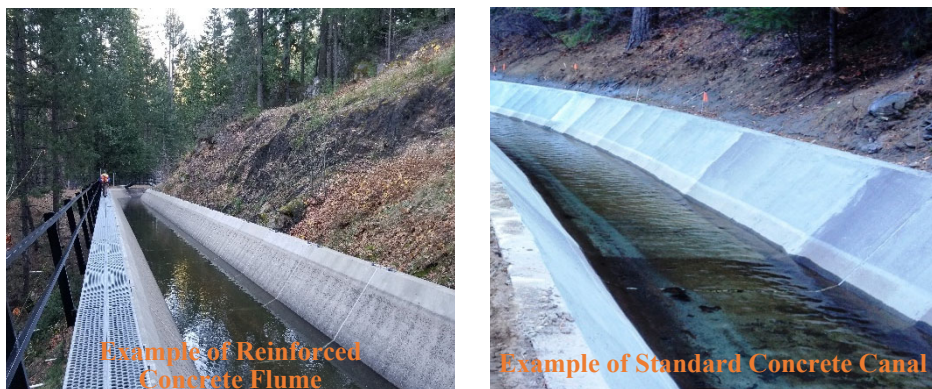
Figure 2-6: Examples of a Reinforced Concrete Flume and Standard Concrete Canal
