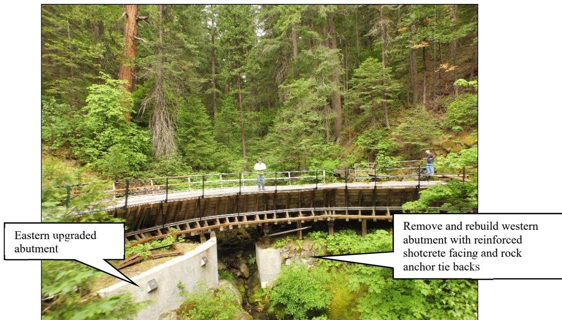
Figure 2-4: Elevated Flume Segment over Bull Creek
