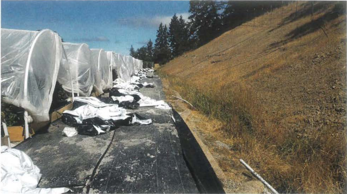
Photograph of the drainage ditch along the northeastern edge of Cultivation Area A. This photograph was taken looking northwest. Note the well vegetated ditch, straw wattles, graveled surface, and weed matting all used to slow and capture surface runoff from the cultivation area.
