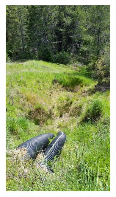
**Photo 5**. View of culverts behind earth dam of Lower Pond and erosion, with Class II drainage below
