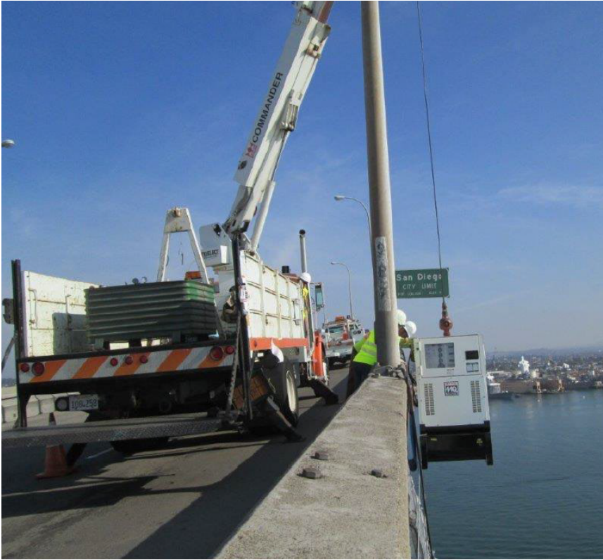
Figure 0-11 Current Generator Access During Maintenance Activities
