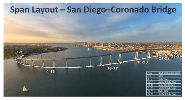
Figure 1-10 Proposed Bay Enclosures of Various Bridge Spans
