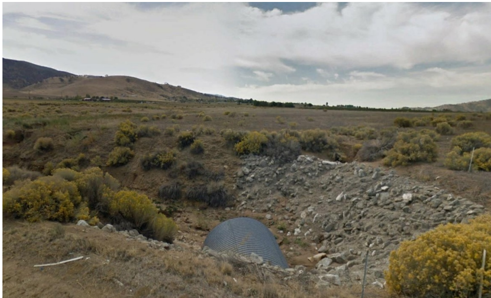
Figure 4: Tucker Rd. Culvert with Concreted Rock Slope Protection. Photo faces southwest from the west shoulder of Tucker Road
