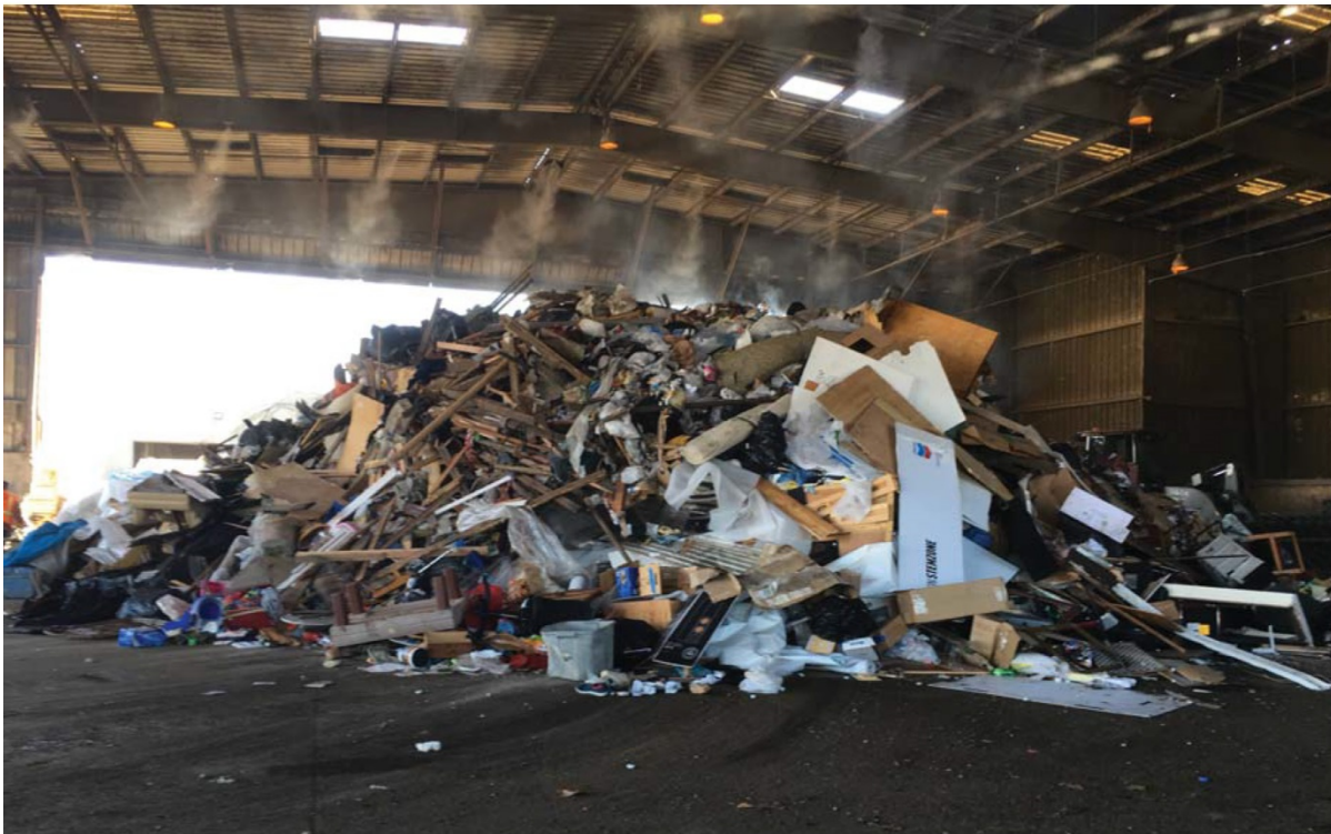
Photo 6: View of municipal solid waste storage area and dust/odor control misting system from tipping floor
