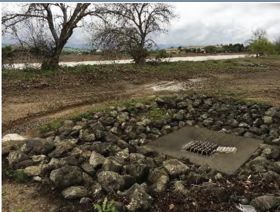
Drainage grate surrounded by riprap rock for excess stormwater flow situated on easterly portion of site
