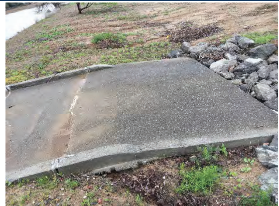
Concrete paved outlet situated along easterly portion of site
