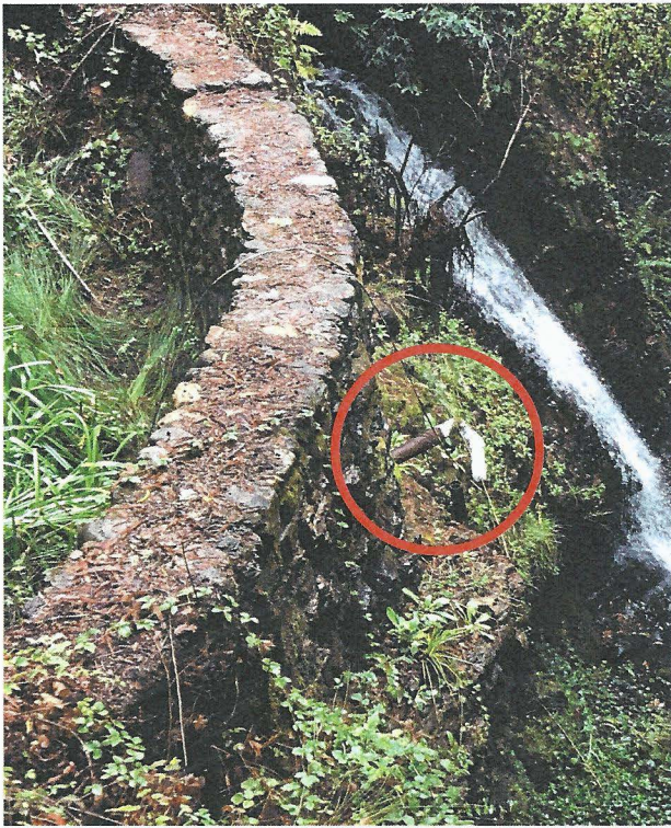
Image #1 (above): Outlet pipe at bottom of the rock-dam reservoir. New pipe to be installed at this point and run down face of cliff. Image #3 (below): Existing puncheon spanning Cascade Creek.
