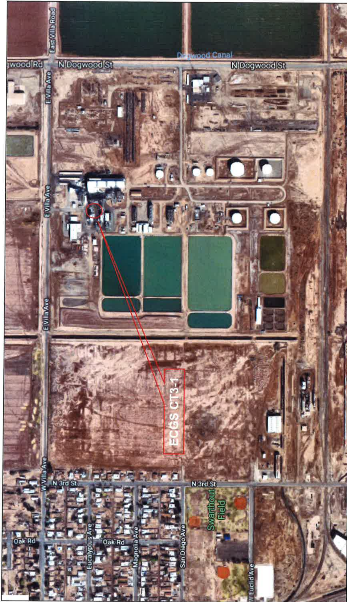
El Centro Generation Station Unit Combustion Turbine 31 Blade Replacement Project
