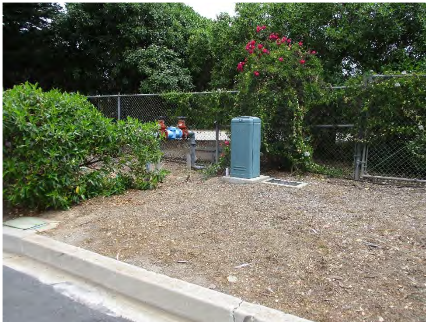
Irrigation Backflow Preventer
