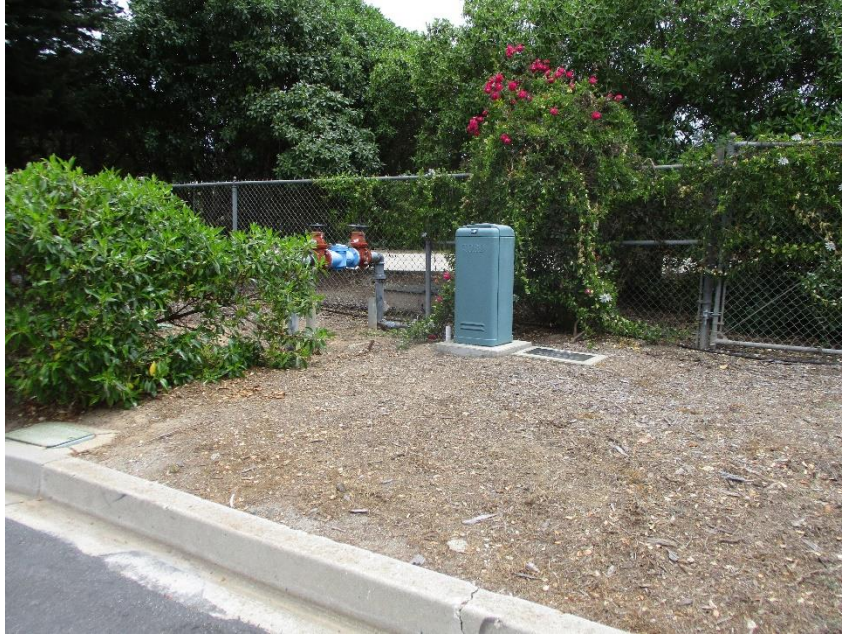
Irrigation Backflow Preventer
