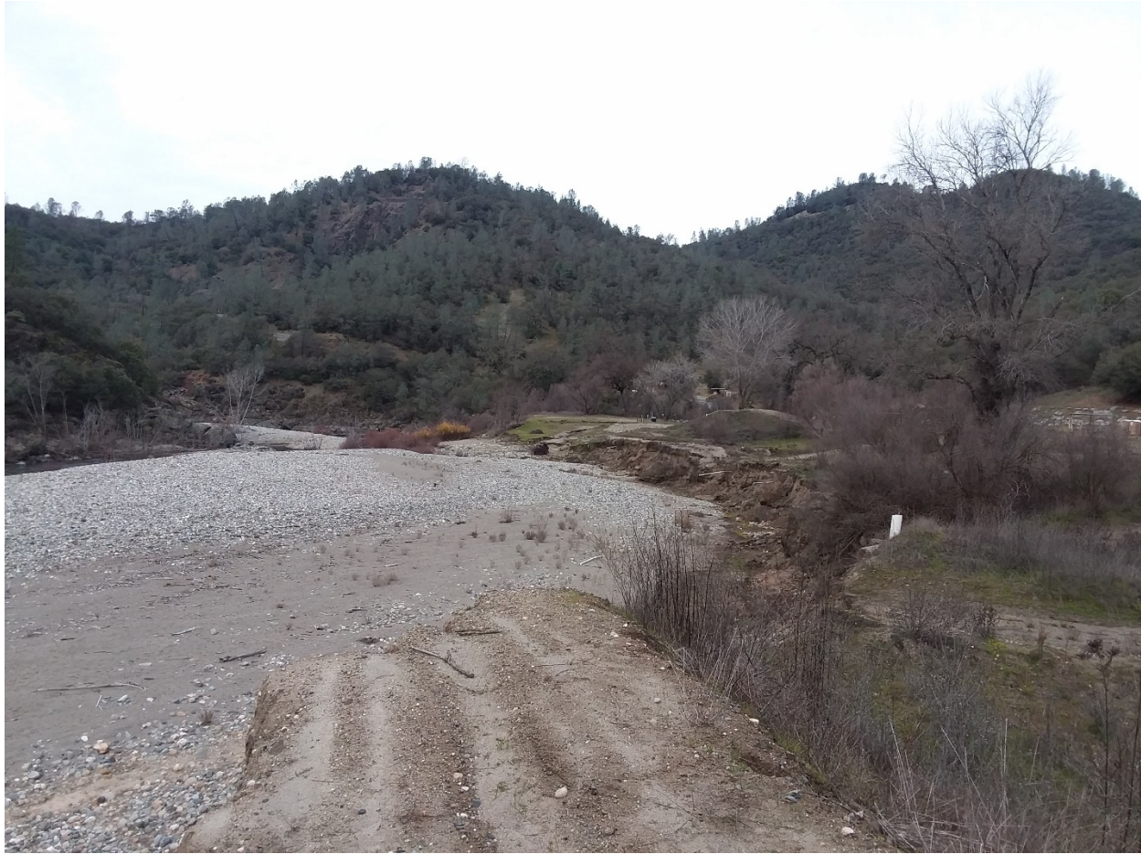
Photo 2. Looking west from the existing MX track. The Middle Fork of the American River is visible in the background to the left. The cut bank caused by high river flows and flooding in early 2017 is visible to the left. A portion of the existing MX track was washed away.
