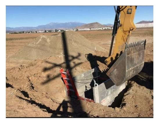
Photo 1 – Looking northeast at DRT-2 and shoring used in all excavations
