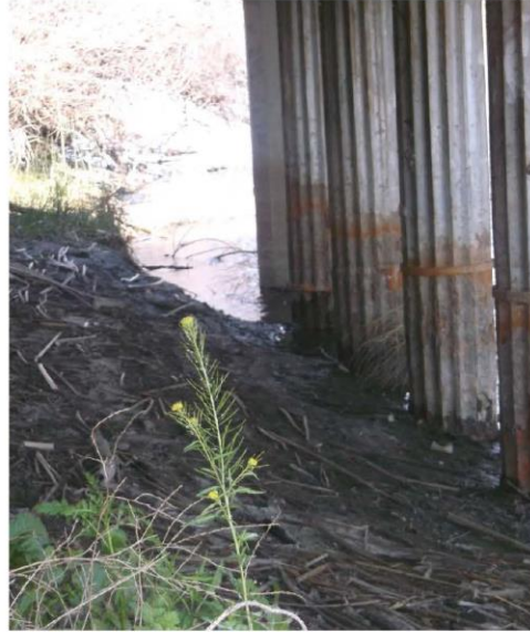
Representative Photo 2: Kings River Bridge with water-stained columns and wrackline of debris, facing north.
