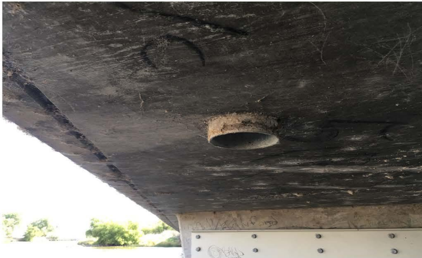
May 24, 2018. Weep hole extending through the deck of the bridge.
