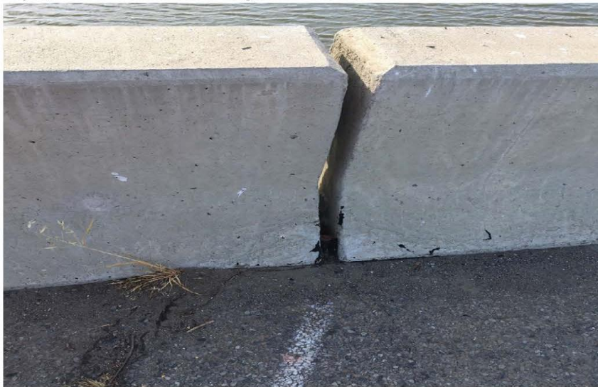
May 24, 2018. View of joint from the top of the bridge. The joint extends through the bridge from the top of the bridge and creates a 1.5" to 2" gap across the underside of the bridge.
