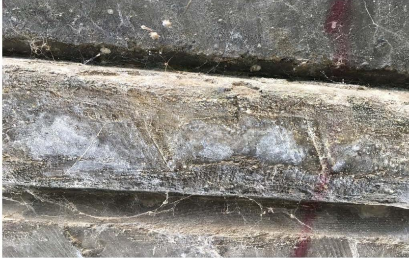
May 24, 2018. Groove extending the length of the underside of the bridge.
