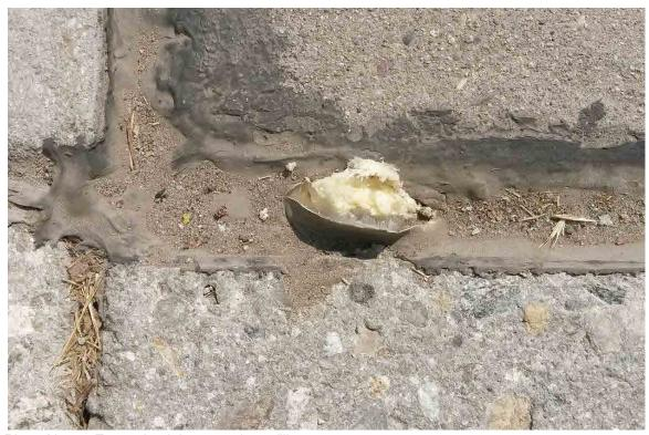
Photo No. 6 Expansion joint spray foam fill
