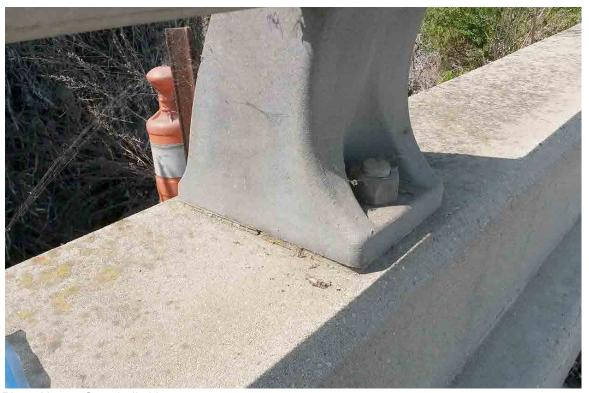
Photo No. 4 Guardrail shims
