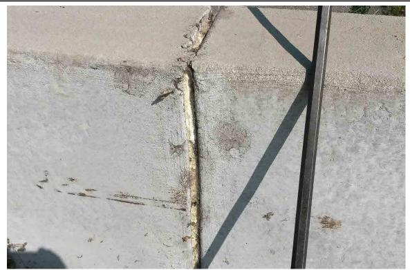
Photo No. 5 Expansion joint styrene fill
