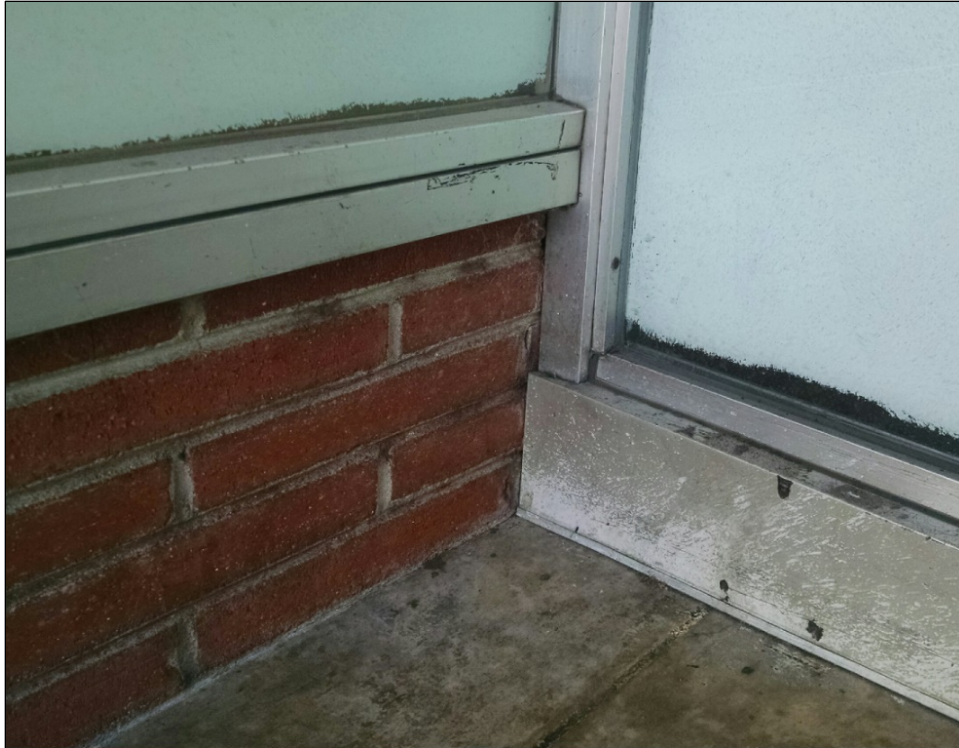
Figure 46. Articulation of rectangular storefront window, brick bulkhead, and door assembly on former Union Hardware building, camera facing north (SWCA, May 5, 2019).
