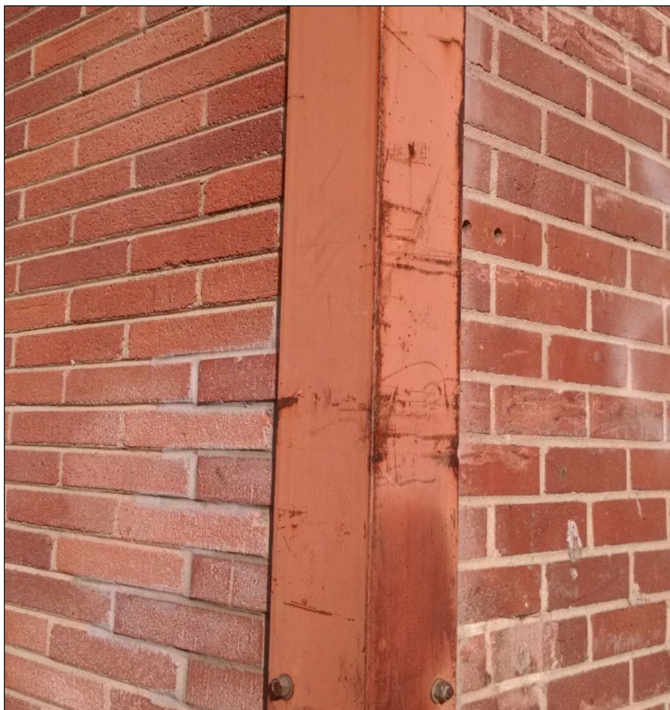
Figure 81. Steel angle bar protecting brick masonry at corner of Marsh Street alleyway behind Rileys building (SWCA, May 5, 2019). Note difference in brick type and dimensions, and in depth of mortar tooling, camera facing west.
