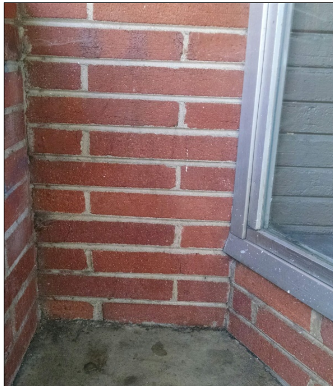
Figure 53. Inner corners of Roman brick masonry between bench and angled display window, camera facing northeast (SWCA, May 5, 2019).
