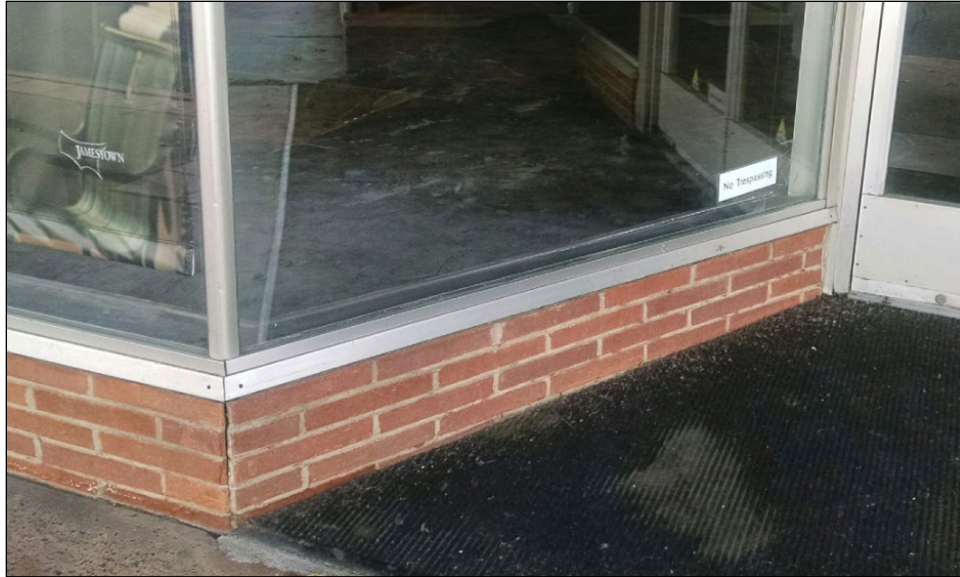
Figure 57. Angled display window at left side of main Chorro Street entrance, camera facing north (SWCA, May 5, 2019). Note gap in brick masonry at exterior corner of bulkhead.
