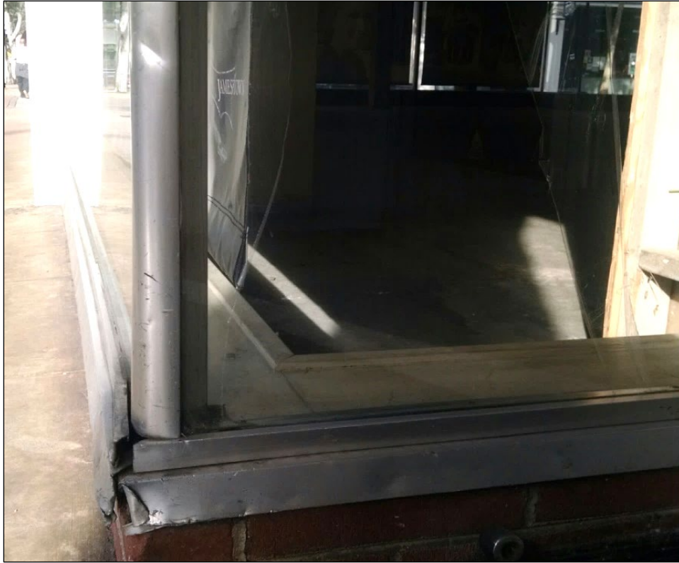
Figure 70. At east end of display window, aluminum frame flares out on top of brick masonry, Marsh Street elevation, camera facing west (SWCA, May 5, 2019).
