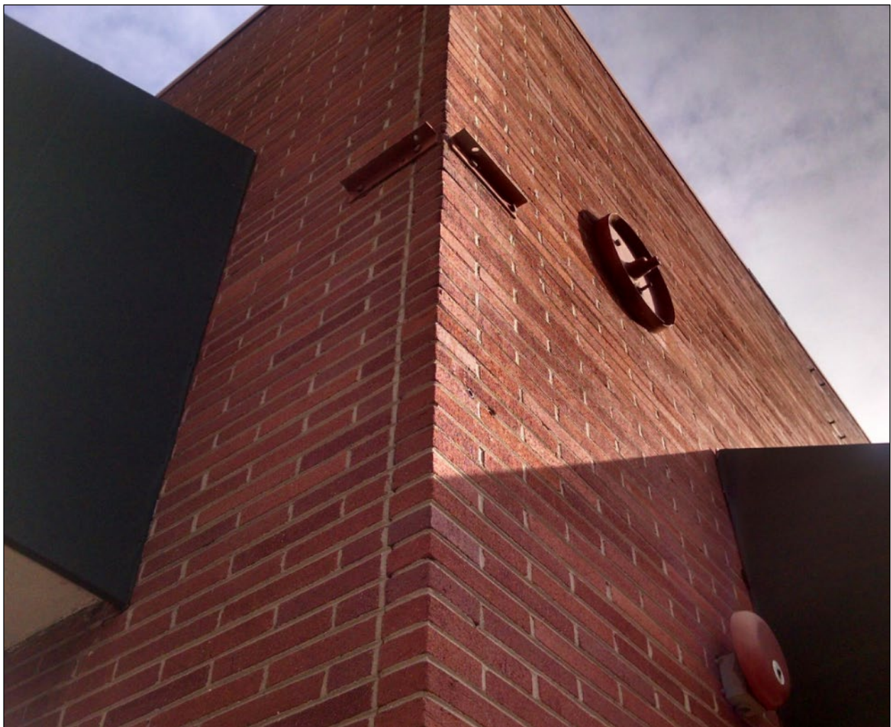
Figure 62. Articulation of Roman brick masonry walls at the corner of Chorro Street and Marsh Street, with brackets that formerly held the vertical Rileys sign and flagpole, camera facing north (SWCA, May 5, 2019).
