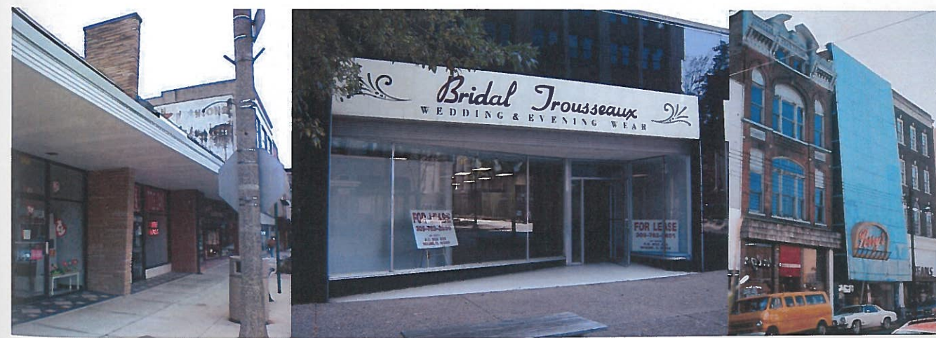
Figure 4: Left, a Freeport, Illinois, angled stone pylon. Center, a Moline, Illinois, example of the common post-war angled open storefront, shown here in structural glass. Right, a much more unusual design angles the entire porcelain enamel facade out from top to base. Left photo: author, center and right photos: IHPA archives
