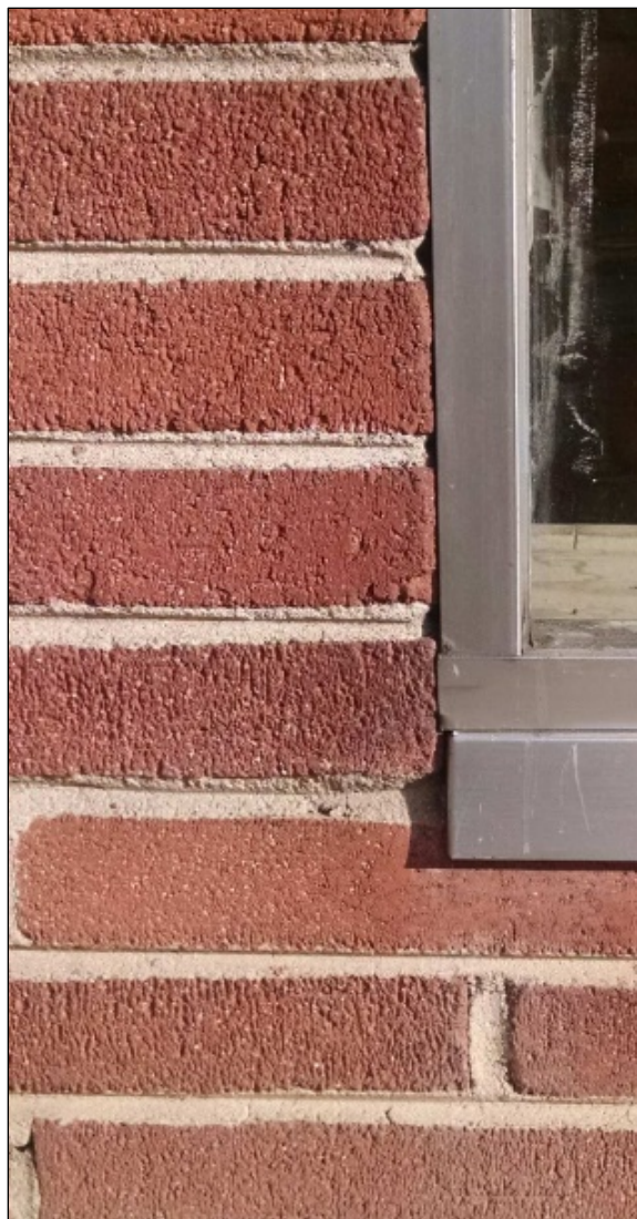
Figure 67. At west end of display window, aluminum frame is flush-mounted in brick wall, Marsh Street elevation, camera facing northwest (SWCA photograph, May 8, 2019).
