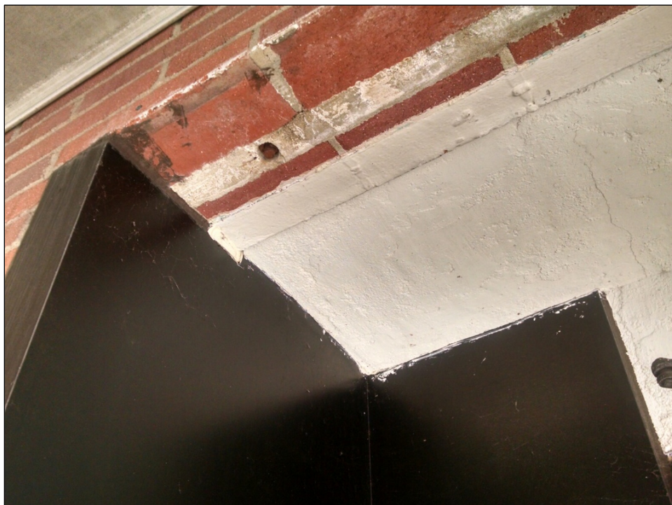
Figure 80. Upper corner of Marsh Street entrance near alleyway, showing where display window was formerly located, camera facing west (SWCA, May 5, 2019).
