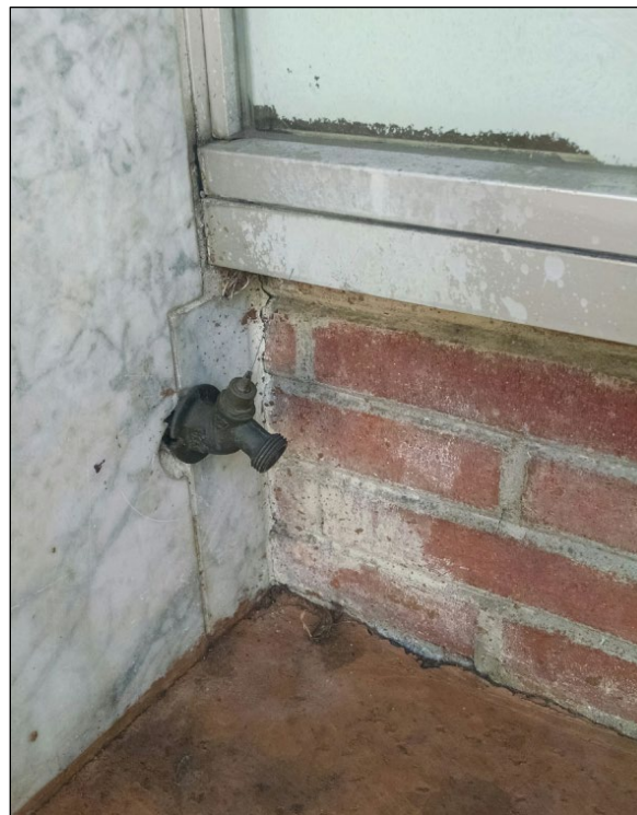
Figure 45. Articulation of marble-clad wall with display window supported on brick bulkhead at left corner of former Union Hardware building, camera facing north (SWCA, May 5, 2019).
