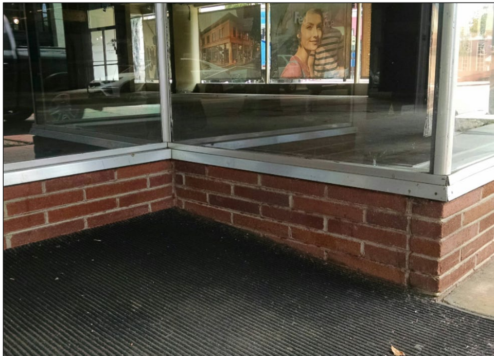
Figure 58. Right-angled corner of display window at right side of main Chorro Street entrance, camera facing east (SWCA, May 5, 2019). Inner corner of bulkhead brick masonry is not integrated into wall plane.
