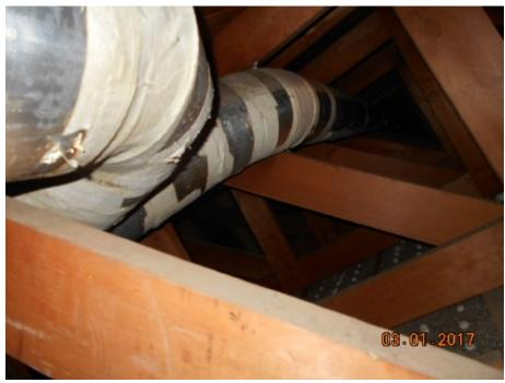
Duct Insulation, Floor 2 crawlspace. Asbestos
