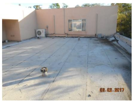
Roof penetration mastics and sealants – asbestos. Lead is present in paint on roof structure stucco.
