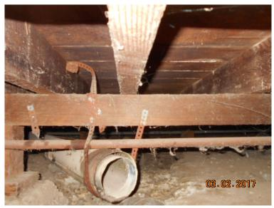
Abandoned duct in sub-floor crawl space
