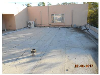
Roof penetration mastics and sealants. No asbestos in main roofing field or in decorative roof shingles.
