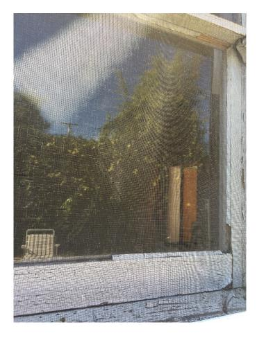
Original white paint on exterior windows and frames is lead-based.
