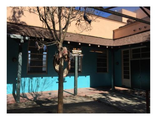
South Exterior Wall. Lead in green paint on posts and double door (only).
