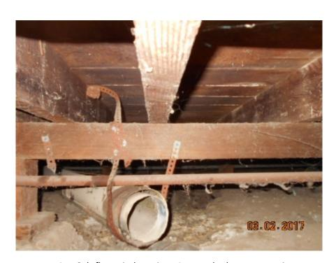
4. Sub-floor air duct pipe. Assumed asbestos wrapping.
