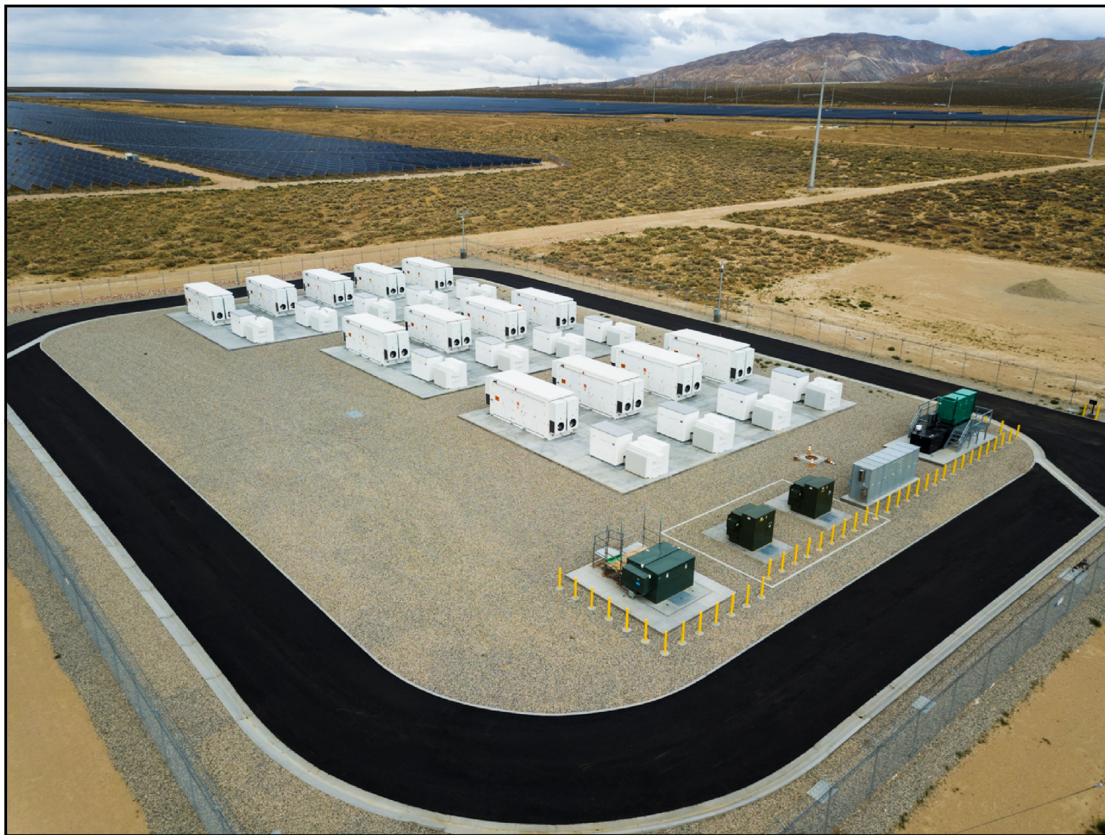
Figure 2-7 Typical BESS Layout
