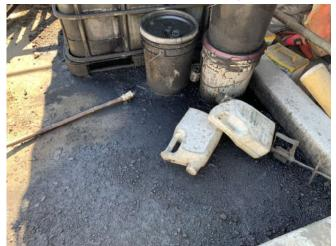
Photo 35: View of the dark staining observed within the secondary containment.
