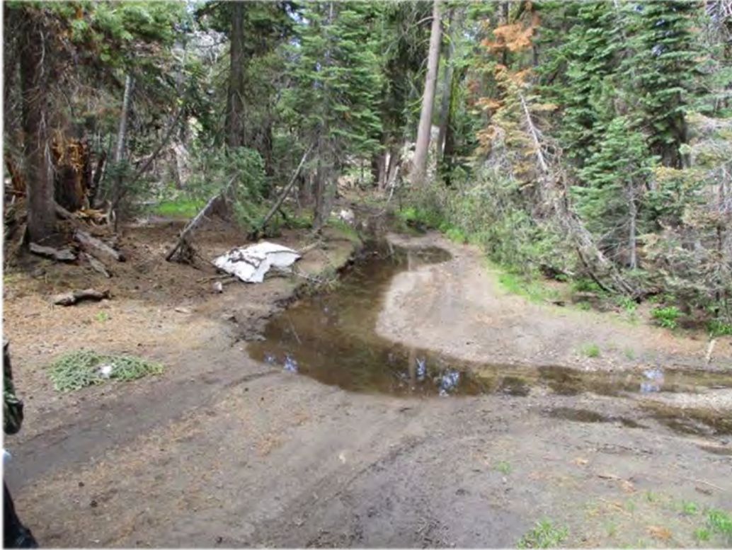
Photo 5. Upper Onion Valley: View to the east of the road that has captured a drainage. July 2019. The proposed road berm would eliminate this occurrence.
