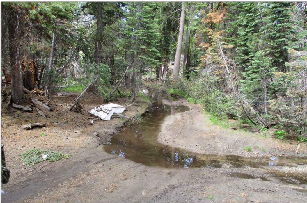
Photo 6. Upper Onion Valley. Stream flow currently captured within road. Road berms will be constructed adjacent to stream channel to direct flows into original channel.
