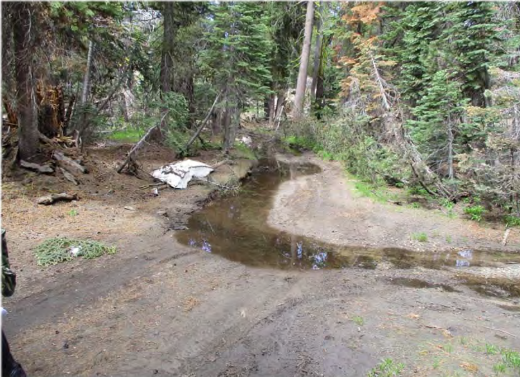
Photo 6. Upper Onion Valley. Stream flow currently captured within road. Road berms will be constructed adjacent to stream channel to direct flows into original channel.
