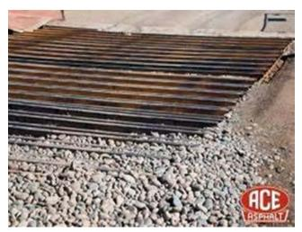
This BMP consists of stabilizing the defined entrance/exit point as well as internal roadways at the facility to reduce exposed sediment becoming airborne and prevent track-out onto public roads by vehicles. Stabilized entrances/exits and vehicle roadways are an effective method for reducing dust and erosion.
