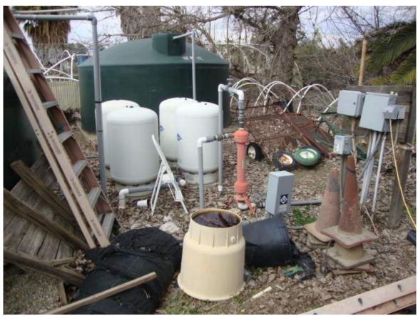
PHOTO 36 VIEW OF THE WATER WELL, BLADDER TANKS, HOLDING TANKS AND FILTERS. PUMP IS ELECTRIC.
