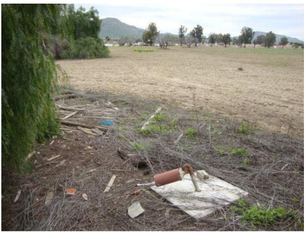
PHOTO 20 VIEW OF A WELL REPORTED IN PREVIOUS ENVIRONMENTAL STUDIES FOR THE SITE LOCATED ON THE WEST SIDE OF THE PEPPER TREES AT THE INTERSECTION OF PARCELS 002, 003, 009 AND 010. THE PIPE IS APPROXIMATELY 2 INCHES IN DIAMETER AND THE CONCRETE IS APPROXIMATELY 2 FEET SQUARE. THE PIPE IS LOOSE AND CAPPED WITH CLAY PIPE AND CONCRETE.
