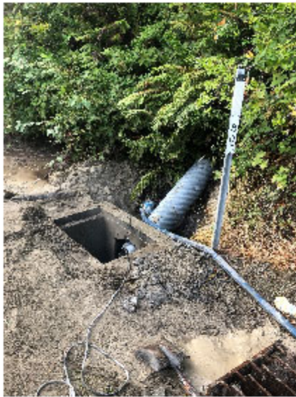
Figure 8. Modification to allow entrapped animals to escape culvert at Butte milepost 47.07, installed 19 September 2019.
