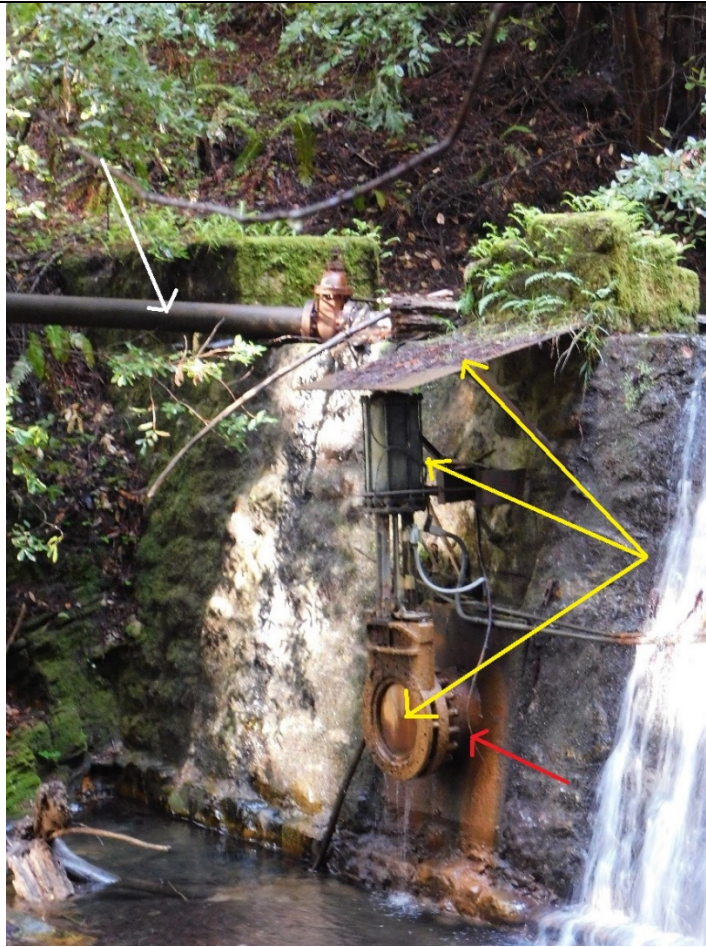
Exhibit 22. West end detail of the Laguna Creek Dam looking northwest showing the non-contributing 1983 sediment bypass valve. The existing gate, actuator, and hood (yellow arrows) will be removed, and a blind flange installed on the end of the bypass pipe (red arrow). The Reggiardo Creek Pipeline (white arrow) crosses the dam to the west of the sediment bypass valve and will not be impacted by the Project (DSCN4851)
