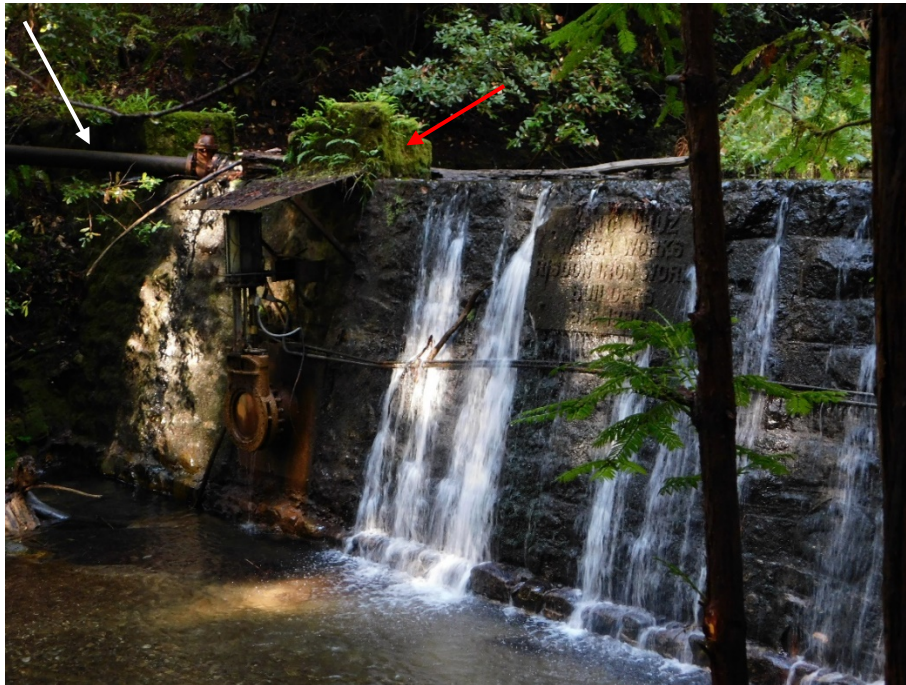
Exhibit 11. Detail of the west side of Laguna Creek Dam showing the masonry column (red arrow) containing the west sediment control bypass valve which separates the two spillways, as well as the Reggiardo Creek Pipeline blow off pipe (white arrow,) view looking northwest (DSCN4853)
