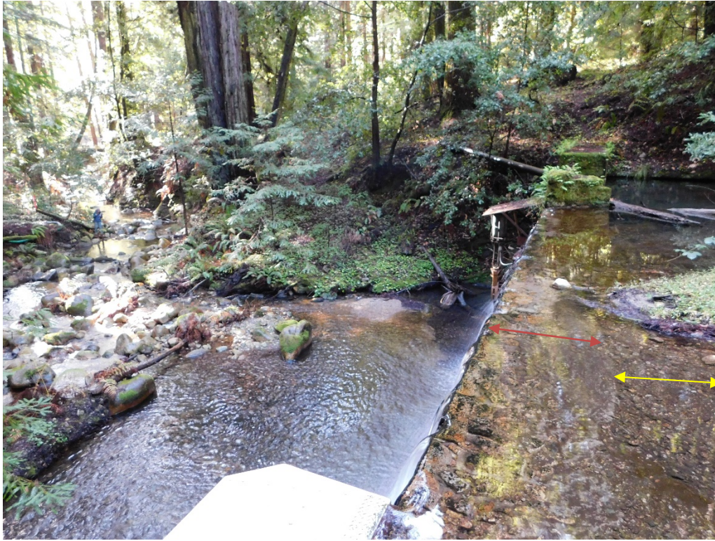
Exhibit 6. The crest of the Laguna Creek Dam (red arrow) submerged in impounded water and sediment (yellow arrow), view looking southwest (DSCN4892)
