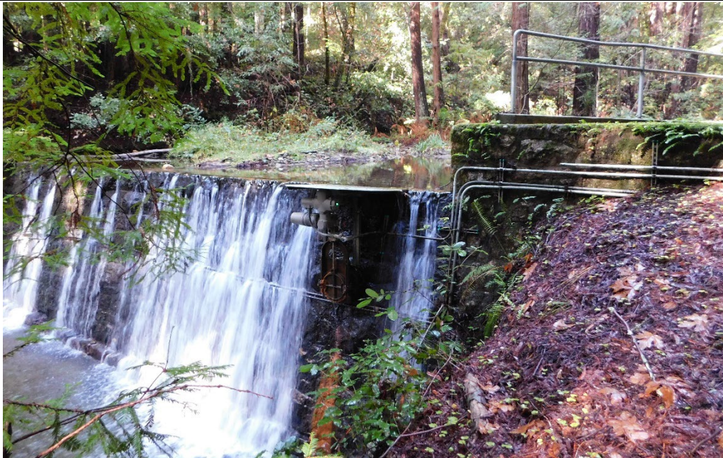
Exhibit 7. Eastern end of the Laguna Creek Dam showing the post-1983 sediment control bypass valve beside the raised corner housing the intake, view looking northwest (DSCN4856)
