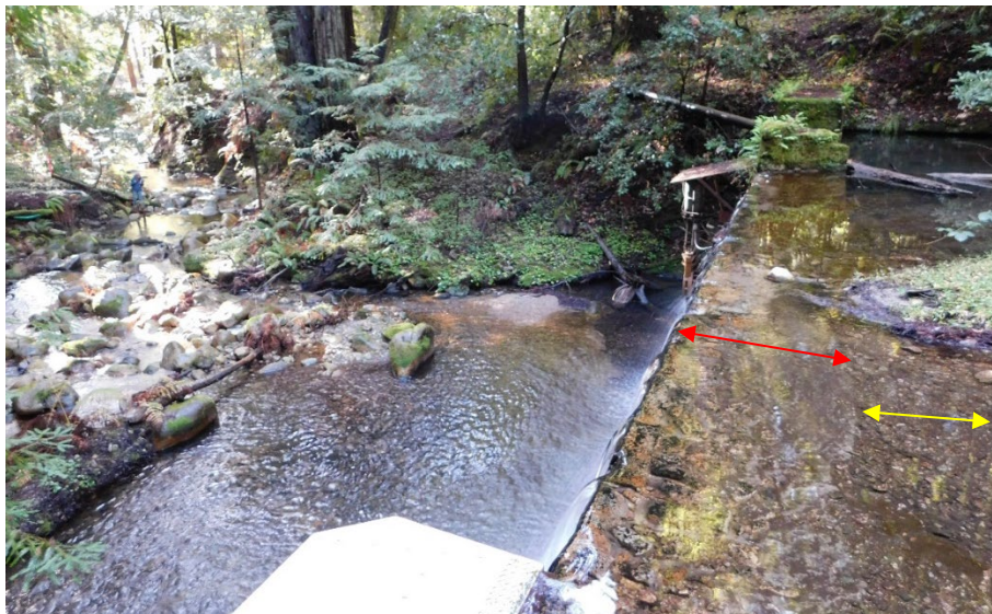
Exhibit 12. The crest of the Laguna Creek Dam (red arrow) submerged in impounded water and sediment (yellow arrow), view looking southwest (DSCN4892)
