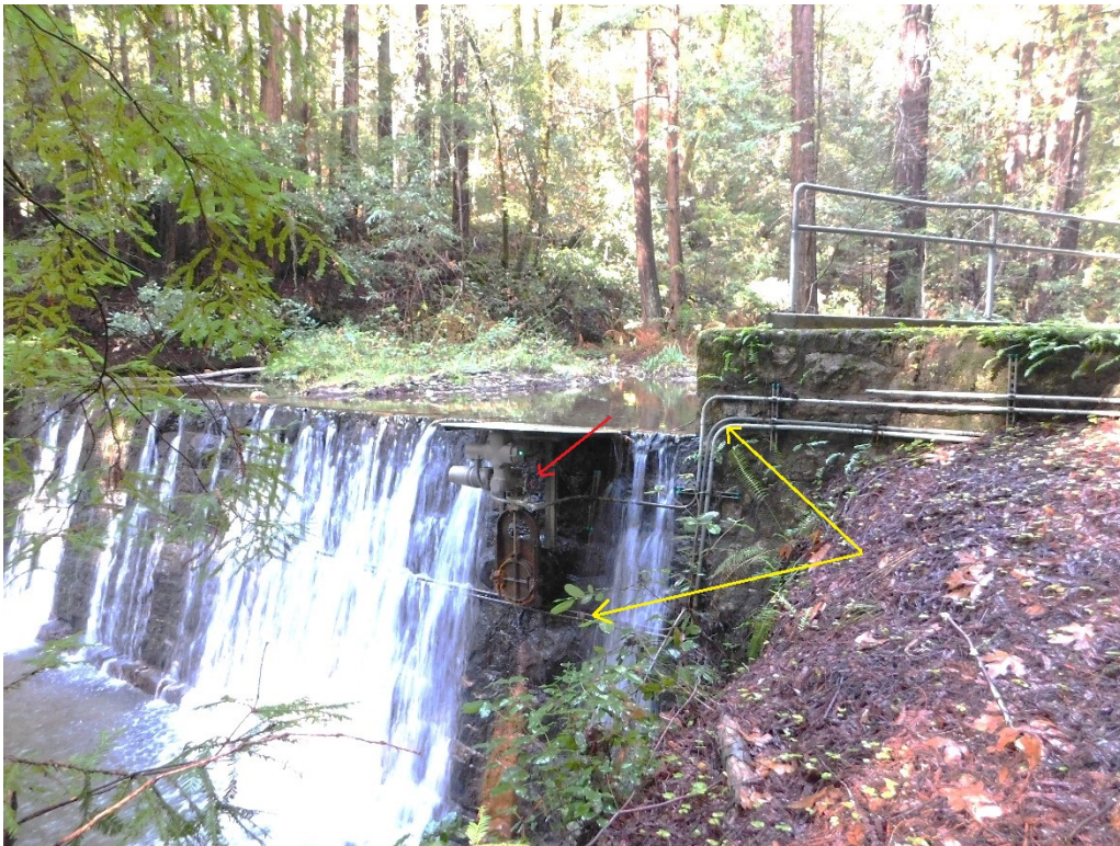
Exhibit 21. East Side of the Laguna Creek Dam showing the non-contributing post-1983 sediment control bypass valve and housing (red arrow), as well as the metal conduit presently attached to the face of the dam (yellow arrows), view looking northwest (DSCN4856)
