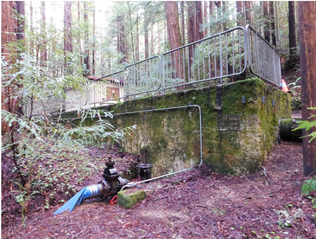
Exhibit 10. Masonry Diversion Flume showing the flume drain (foreground) and the head of the Transmission Pipeline (right). Chlorination Station building in background, view looking northeast (DSCN4823)
