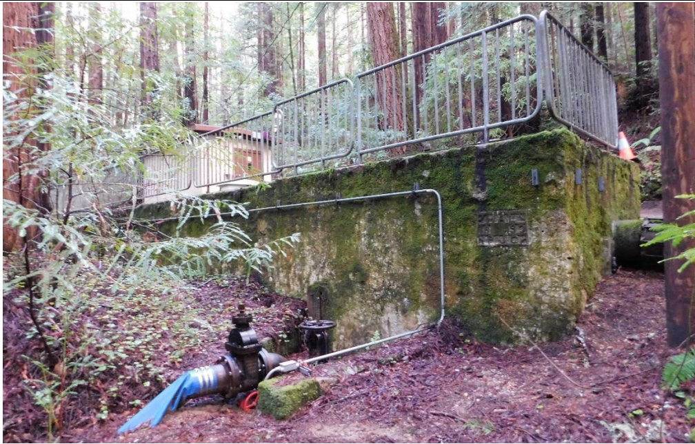
Exhibit 16. Masonry Diversion Flume showing the flume drain (foreground) and the head of the Transmission Pipeline (right). Chlorination Station building in background, view looking northeast (DSCN4823)
