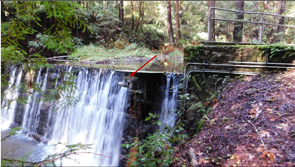
Exhibit 13. Eastern end of the Laguna Creek Dam showing the post-1983 sediment control bypass valve (red arrow) beside the raised corner housing the intake, view looking northwest (DSCN4856)
