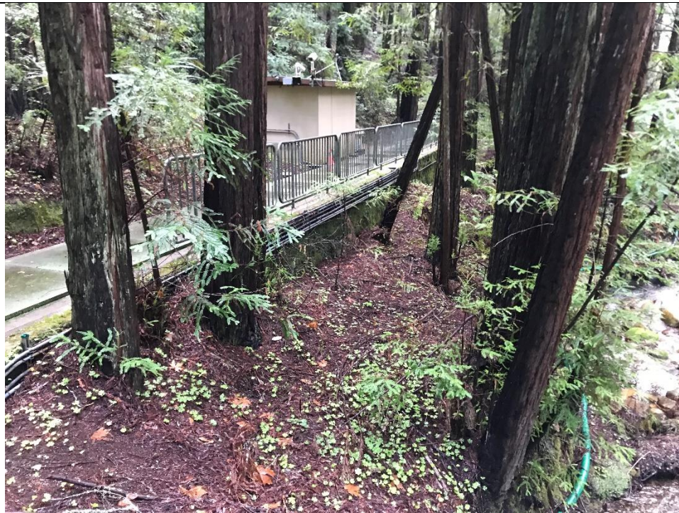
Photo 6: Existing control building and diversion flume. Foreground would be the approximate location of the riprap apron and shows the few redwood trees to be removed. View looking southeast.
