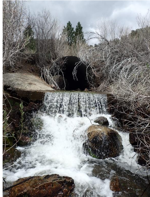
Culvert and fish barrier on By-Day Creek at Buckeye Road
