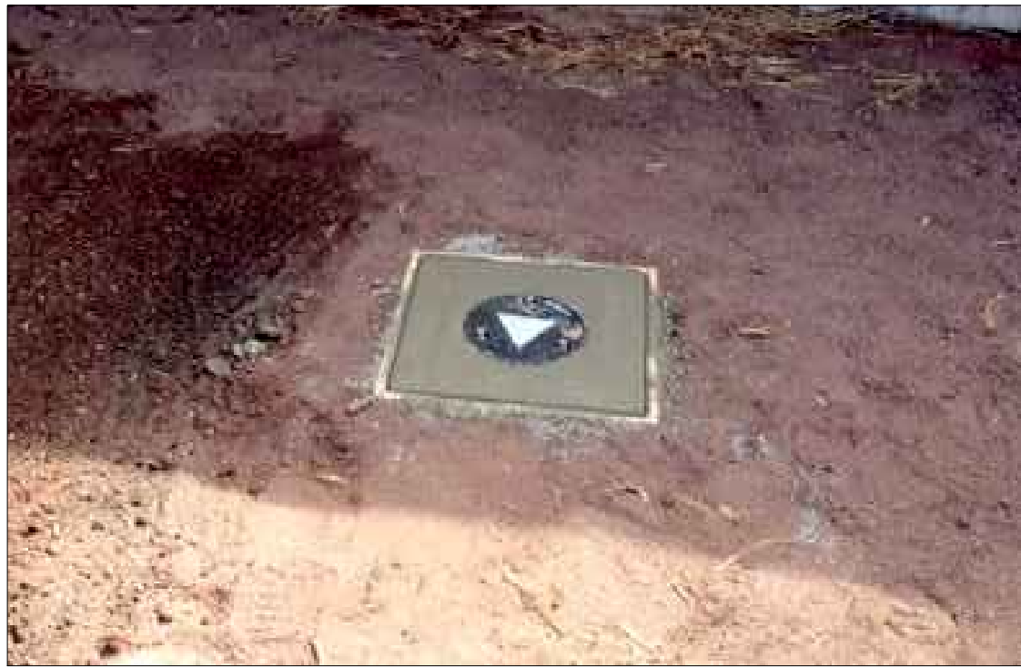
AIR SPARGE WELLHEAD (TYPICAL)
