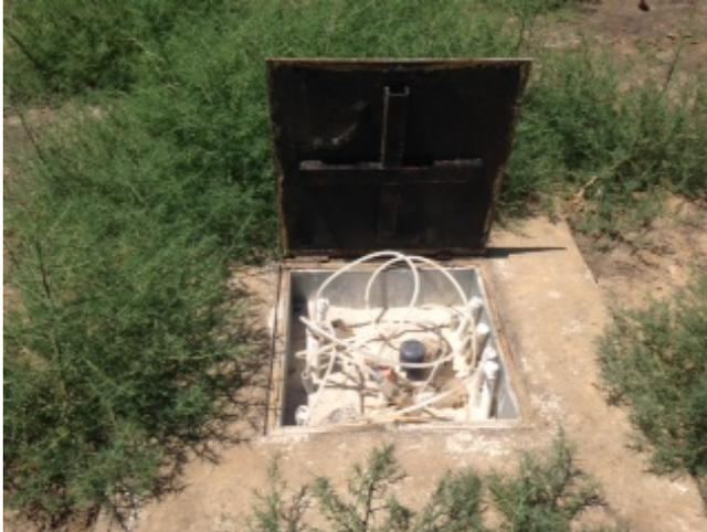
11. Western Parcel. Vault containing nutrient injection ports, vapor recovery well, and monitoring well.
