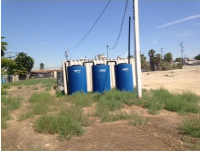
5. Western Parcel. Carbon tanks used for hydrocarbon vapor recovery
