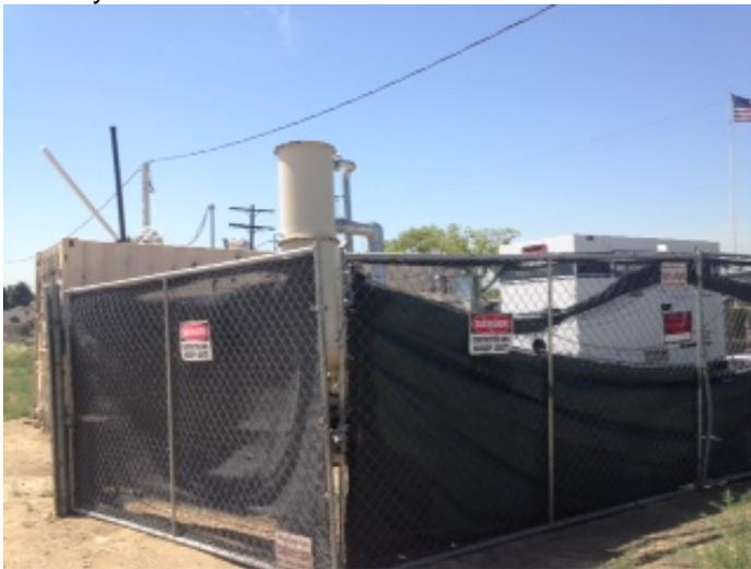
7. Western Parcel. Fenced area containing oxidizer used for hydrocarbon vapor destruction
