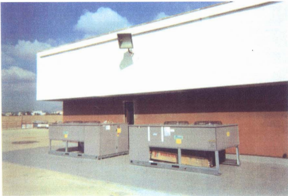
2. View of the second floor. There are two brand new HVAC units located on the roof of the second floor. The old system was abandoned in place.
