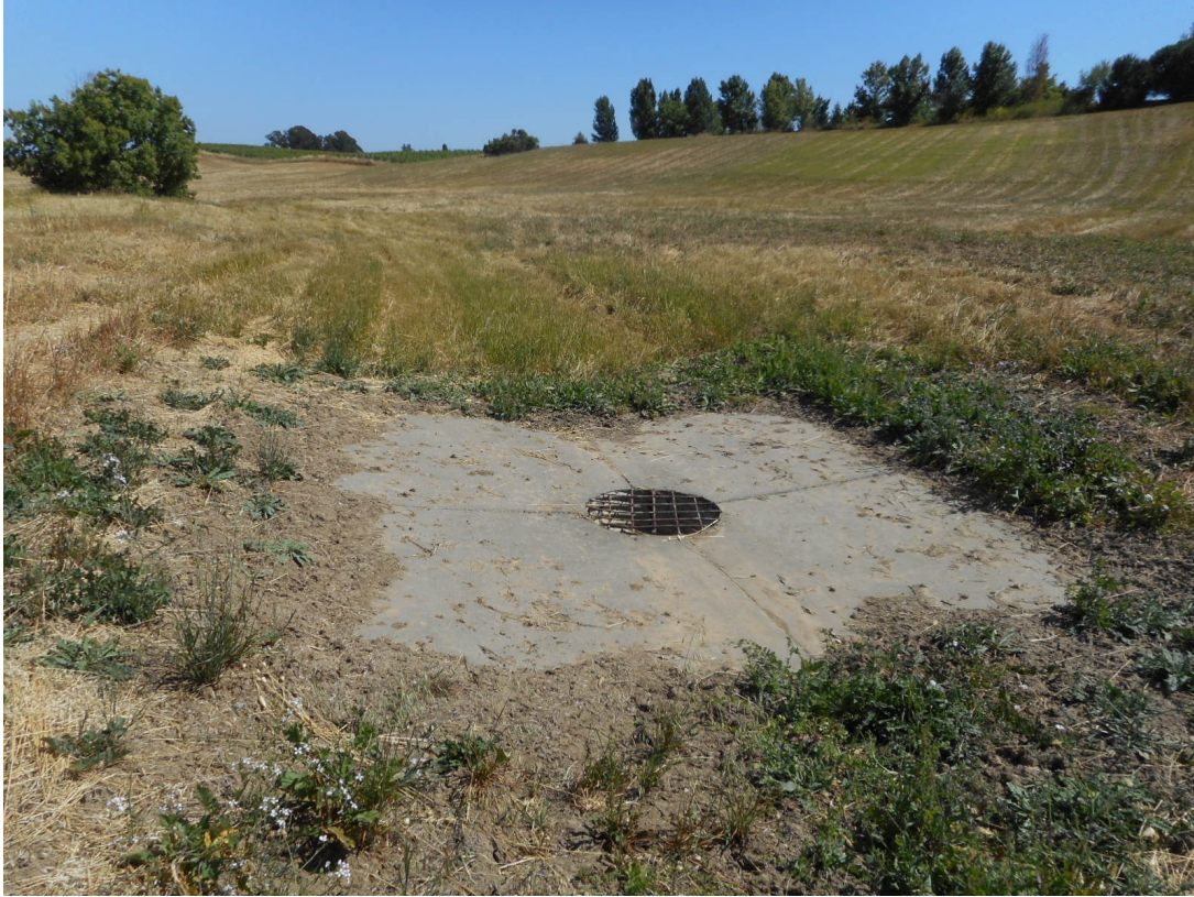
Photo illustrating drop inlet structures along Drainage A.
