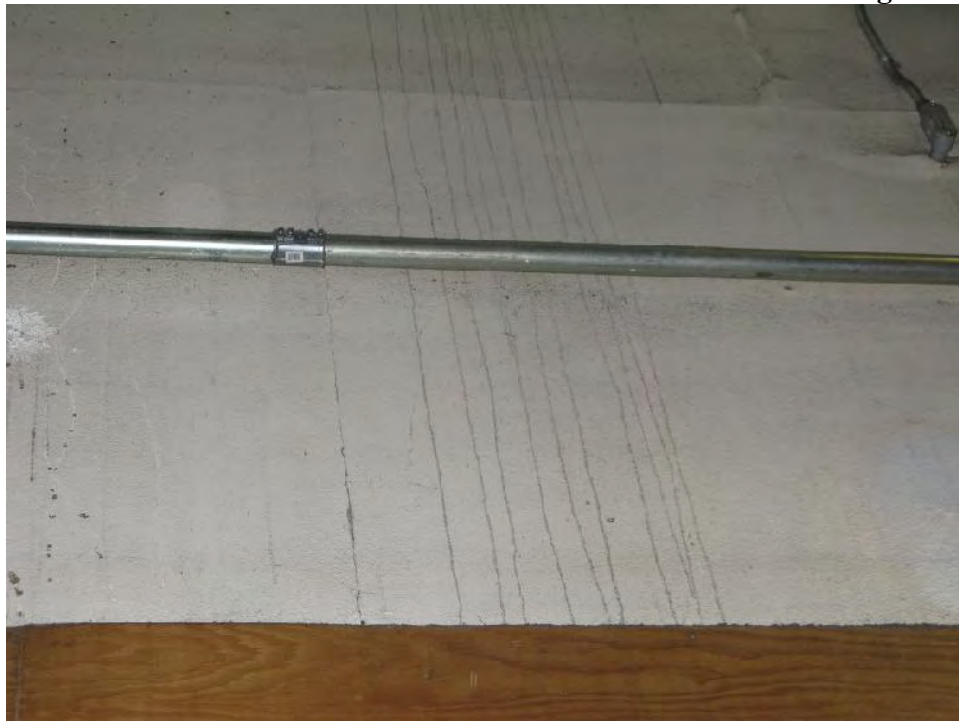
Water Stains on Concrete Wall from Condensation in Cold Storage Area
