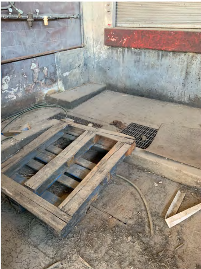
Floor Drain in Truck Ramp
