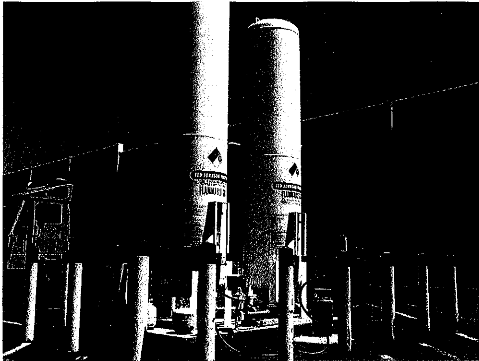
Photo #23 Above-ground propane gas tanks
