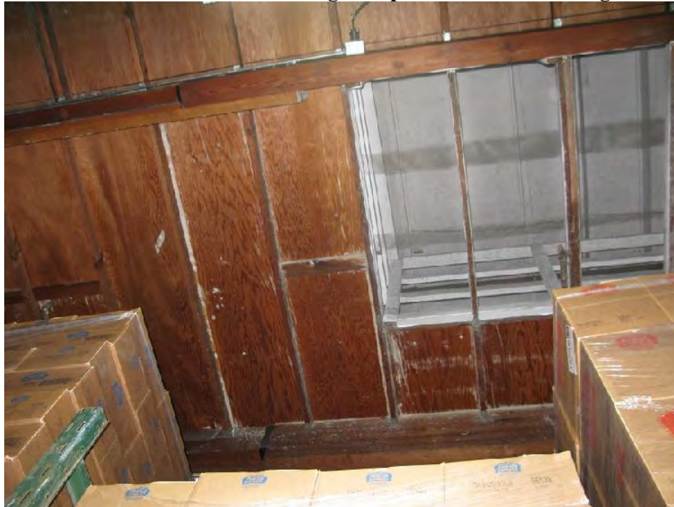
Re-Occurrence of Mold on Ceiling Components in Cold Storage Area
