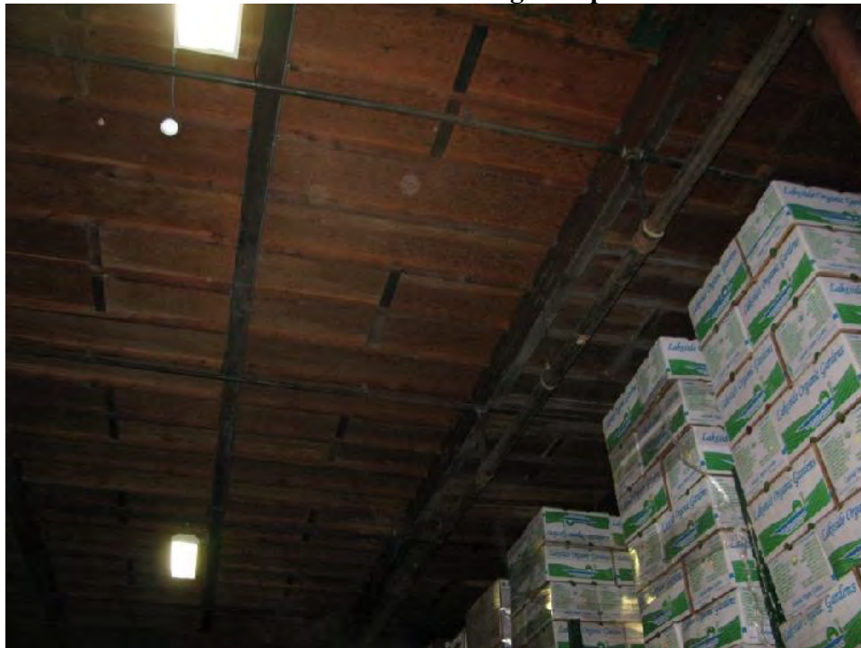
Re-Occurrence of Mold on Wood Ceiling Components Above Boxes
