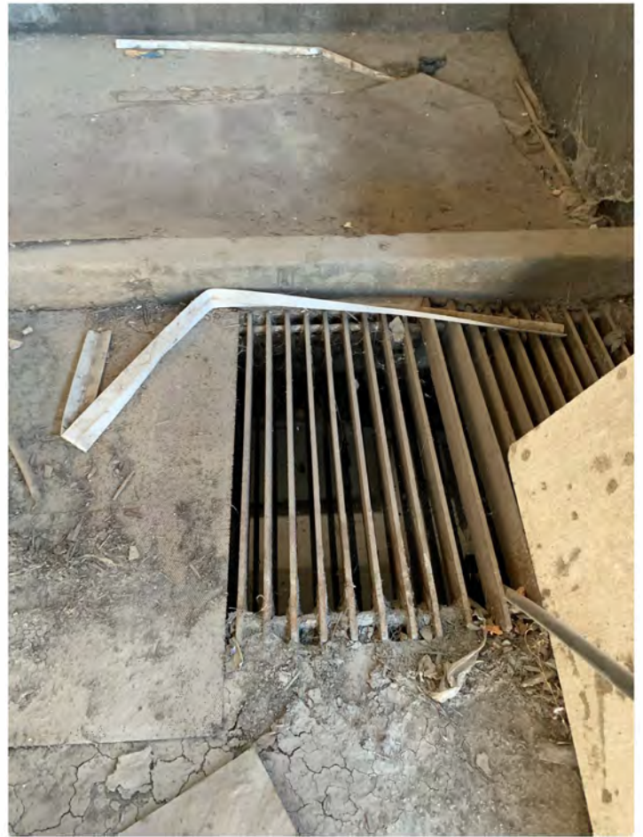
Floor Drain in Truck Ramp
