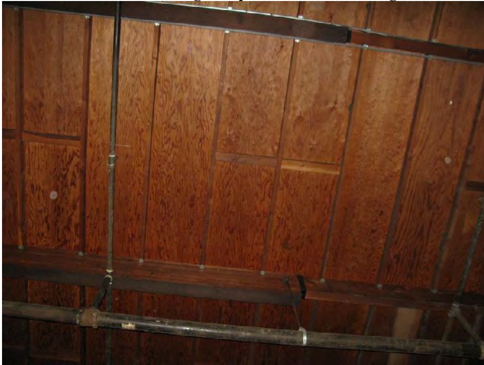
Cleaned Wood Ceiling Components in Cold Storage Area
