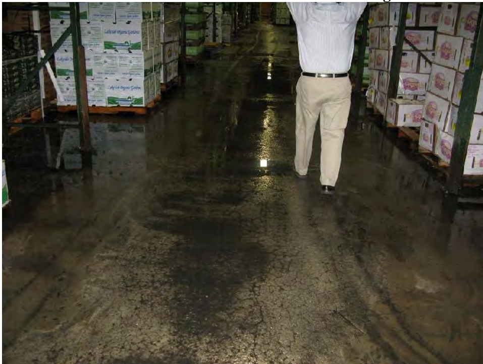
Puddled Water on Concrete Floor of Cold Storage Area
