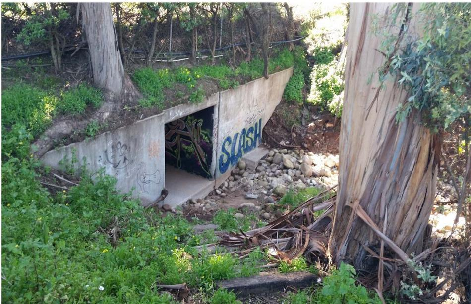
Garrapata Creek exits the Site at the south property boundary, where it flows through this cement box culvert under Highway 101.
