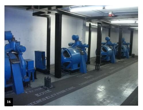
Overhead traction elevator equipment
